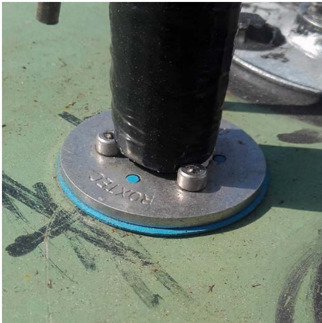
The Roxtec SPM seal installed onboard the barge-pontoon.
